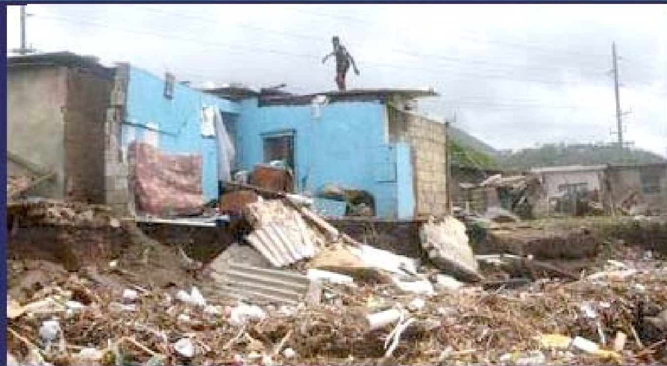
Homeowner surveying the damage.
